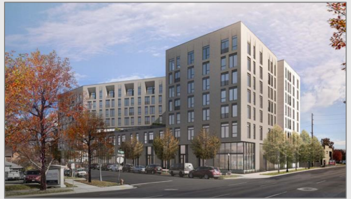
The HEarth, 163 apartment units, 8 stories, 183 parking spaces Photo courtesy Design Review Submittal
