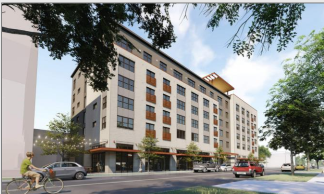
6 stories, restaurant 1 st floor & 114 apartment units Photo courtesy of Design Review Submittal & Pivot North
